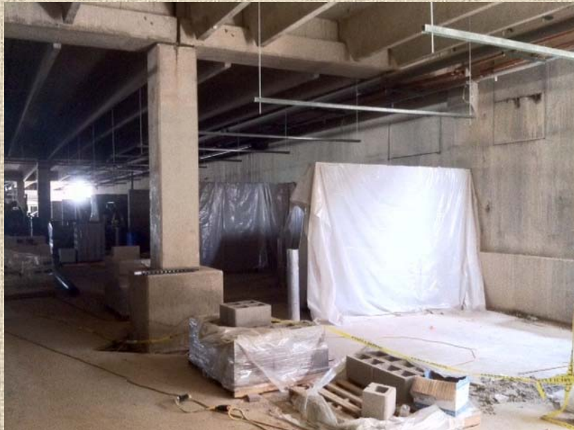
Equestrian Multi-Purpose Facility - Wash Racks
