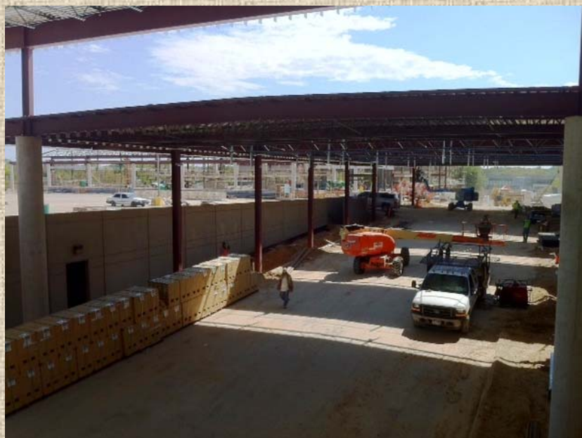
WR Watt Drive Canopy - south side
