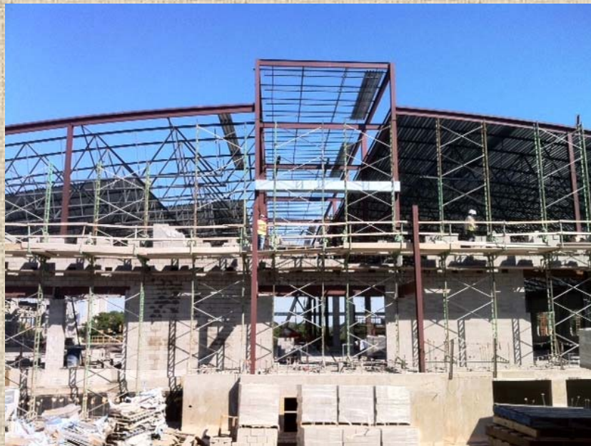
Equestrian Multi-Purpose Facility - West Face
