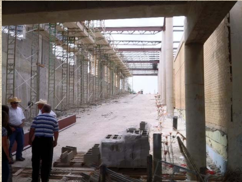
Ramp from Lower Level to WR Watt Drive
