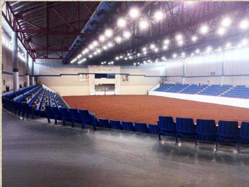
John Justin Arena with new Footing
